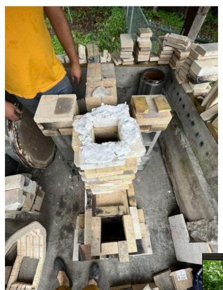
Using pieces of kiln shelf, some split bricks and kaowool, we shimmed the supports to place the kiln bottom.
