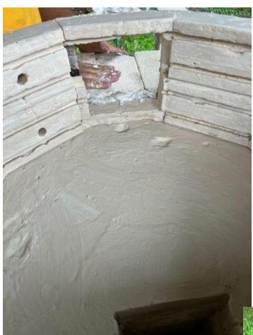
A 7"x7" hole should be cut in one of the sides of the bottom most section of the kiln body. You may need an angle grinder or dremel to cut through the metal of the kiln. Leave a strip of the metal intact on the top and bottom of the hole. Any places with crumbled brick were filled in with Kaowool.
